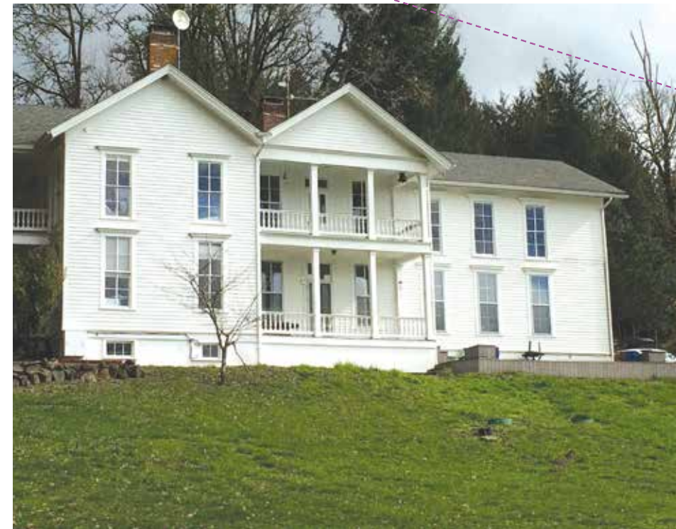
This stately home is perched atop a hill overlooking Plas Newydd Farm. The house is on the National Register of Historic Places as the Columbia Lancaster House. It now serves as the headquarters for Plas Newydd LLC and its 12 employees.
